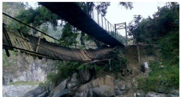
Fig. 2 The old bridge and the new one.
