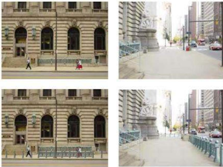
Sensitivity to context is crucial when introducing new security elements, particularly where historic buildings are concerned. Existing building features and materials (top) should inform the design and placement of new security elements (bottom). A kit-of-parts approach can be useful in such cases, to facilitate consistent implementation over time.
