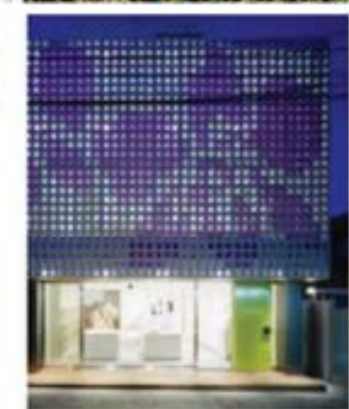
THE BATIK PATTERN MAKES A NICE CULTURAL REFERENCE AND SCREENS THE BUILDING FROM WESTERN SUN EXPOSURE
