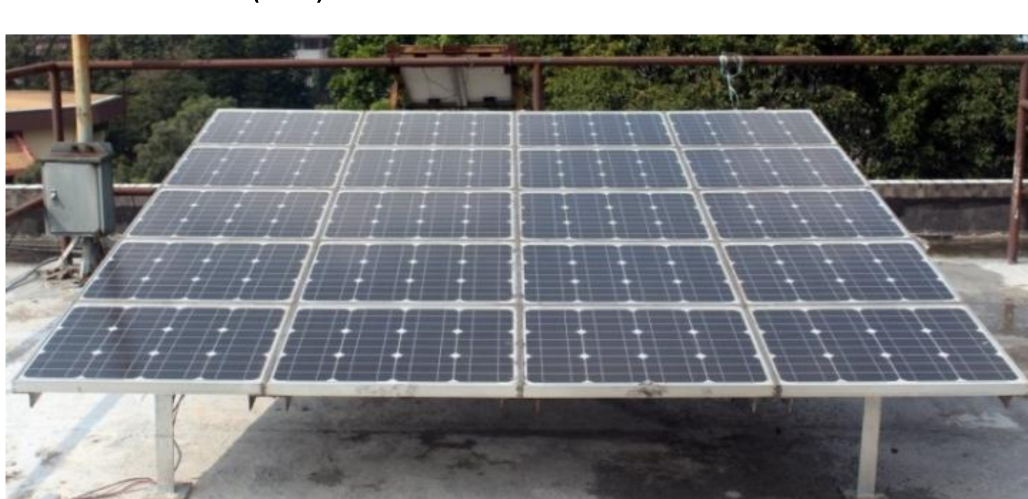
Figure 2. One kWp on-stand PV system at 4 th floor PAU ITB building
