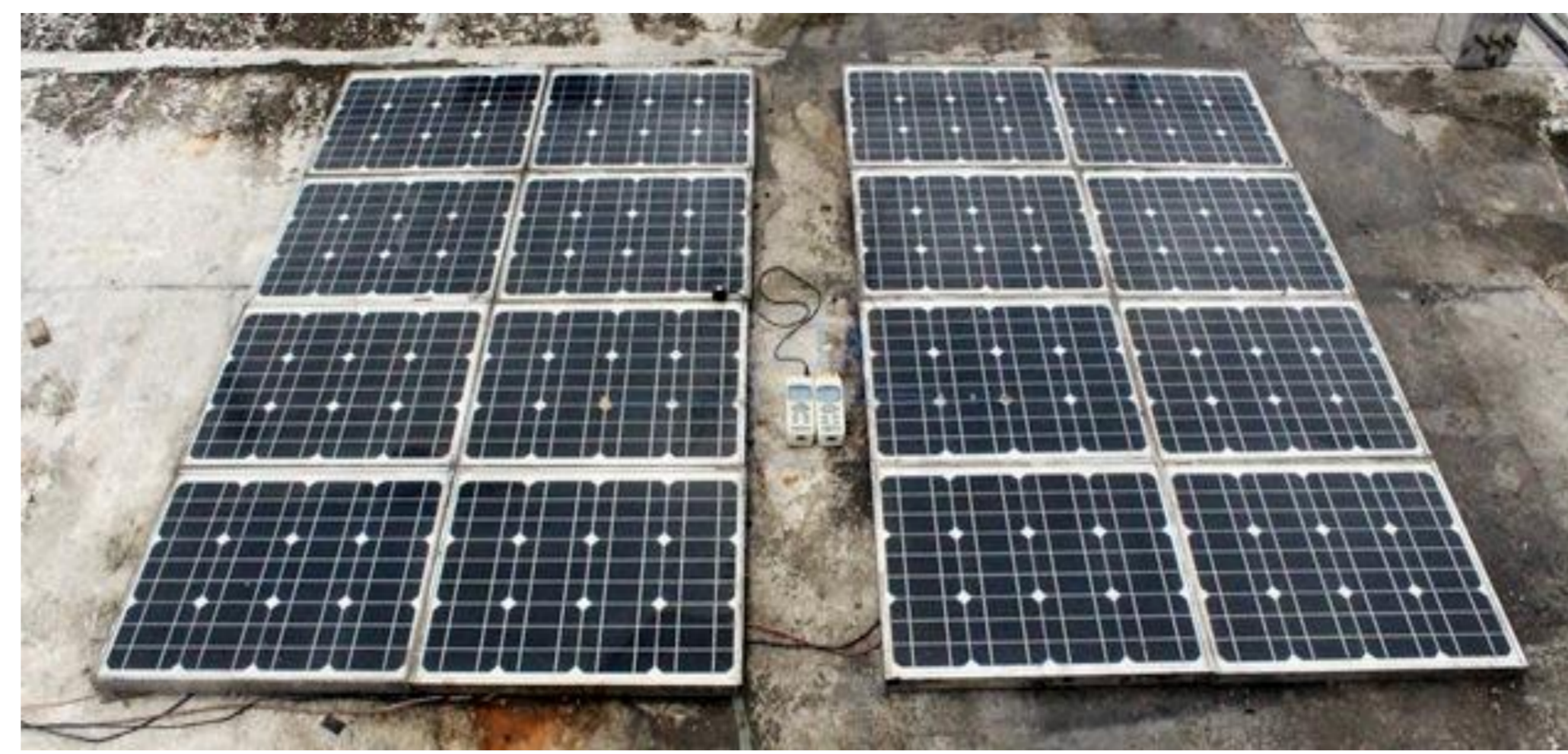
Figure 3. 0.8 kWp on-roof PV system both in on-grid and off-grid PV system
