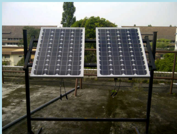
Figure 1. Installation of PV panels outdoor
