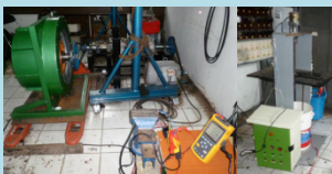
Installation of electrical PMG performance testing
