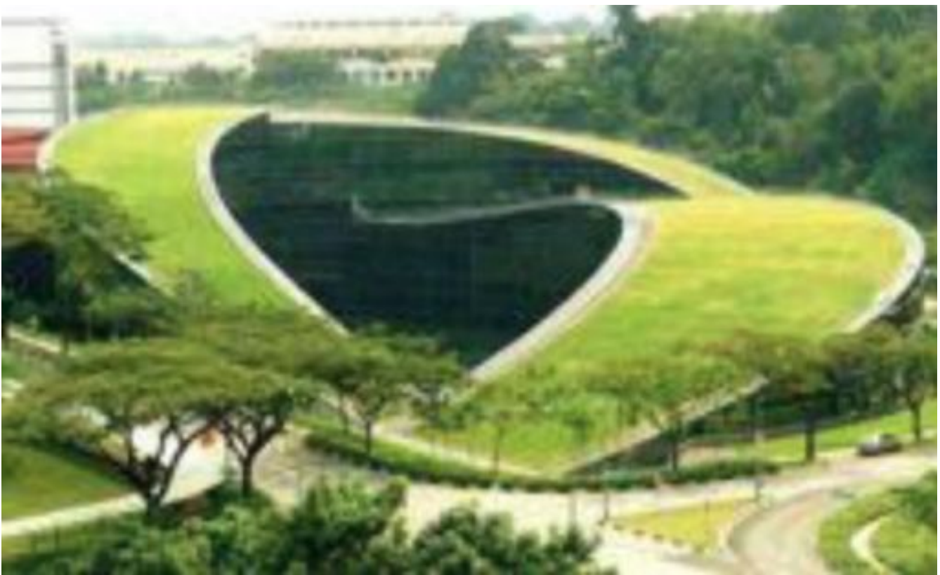
Gambar 7 - Contoh Green building di Nanyang Technological University, Singapura (Sumber: http://www.inhabitat.corn/2008/01/23/amazing-green-roof-art-school-in-singapore )
