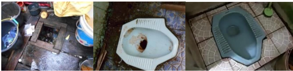
Figure 2. Type of used toilet (a) Hole in the floor (b) Fabricated toilet with broken flush (c) fabricated with good system.
