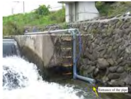
Figure 3. Main pipe velocity of pipe-type fishway Figure 4. Install to Fukano weir in the Kii river
