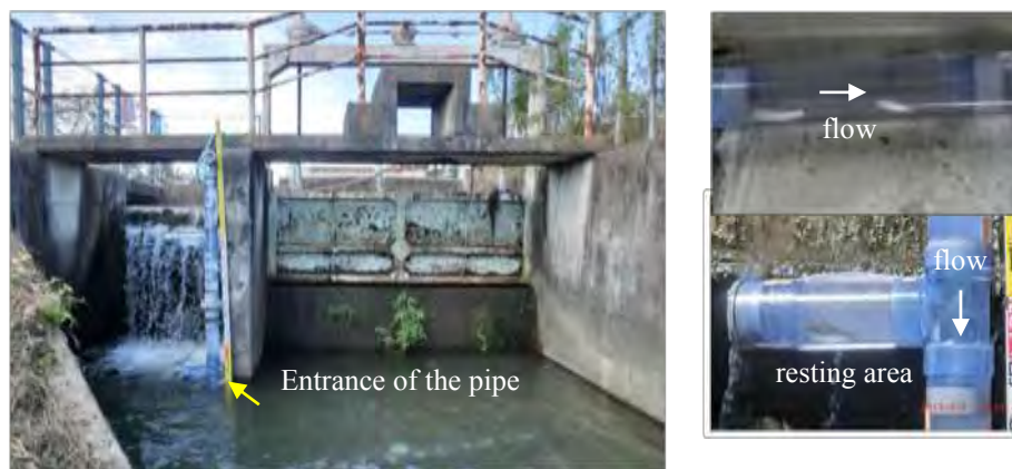
Figure 6. Installing pipe-type fishway to the irrigation system without fishway
