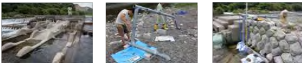
(a) Pool-and-weir fishway (b) Assembling of the fishway (c) Installed pipe-type fishway
