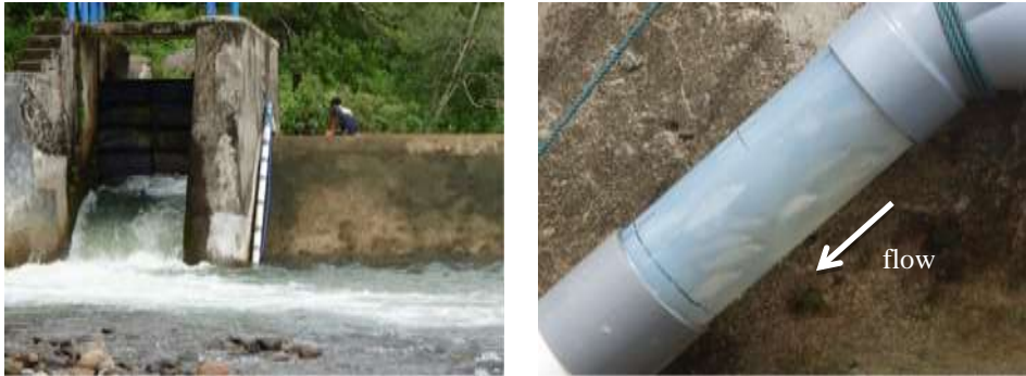
Figure 1. Pipe-type fishway at Parak Buruk Weir in the Kandis River
