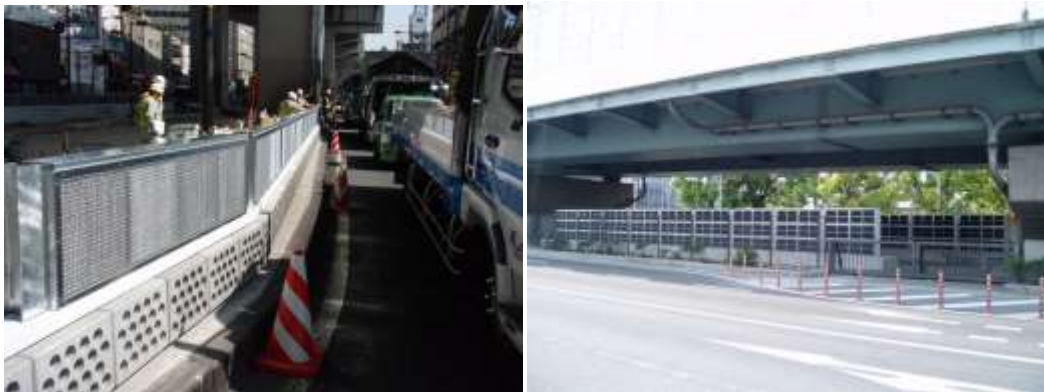
Fig. 5 Installation of ACF fence at the national highway route 43 in Osaka
