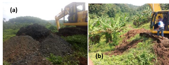
Fig 2. Sampling (disturbed); (a) subgrade soil under zone 1, (b) soil outside the zone of landfills.
