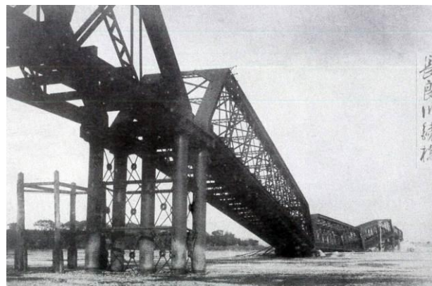
Figure 2. Fall of Nagara-gawa River Iron Bridge (Source: Photo book of the Noubi Earthquake [8] )
