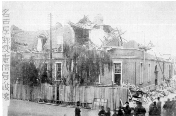
Figure 3. Damage of Nagoya Postal Telegraph Office (Source: Photo book of the Noubi Earthquake [8] )
