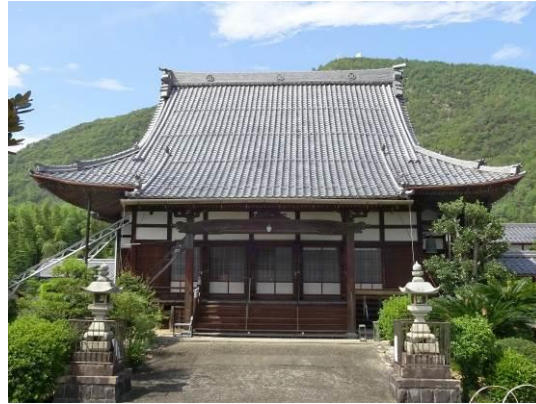
Figure 8. Main Hall at Shinryu-ji Temple
