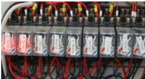
Gambar 23. Relay solenoid valve 1 & 2 ON
