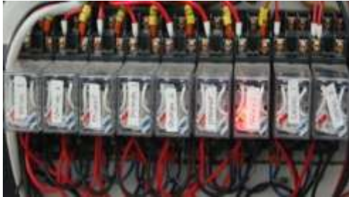
Gambar 28. Relay solenoid valve (SV-3) ON
