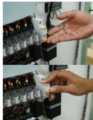
Gambar 16.. MCB (Mini Circuit Breaker)
